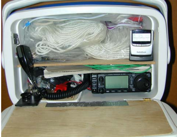
Photo: Fully stocked radio system including solar panel, antenna, and pulleys.
